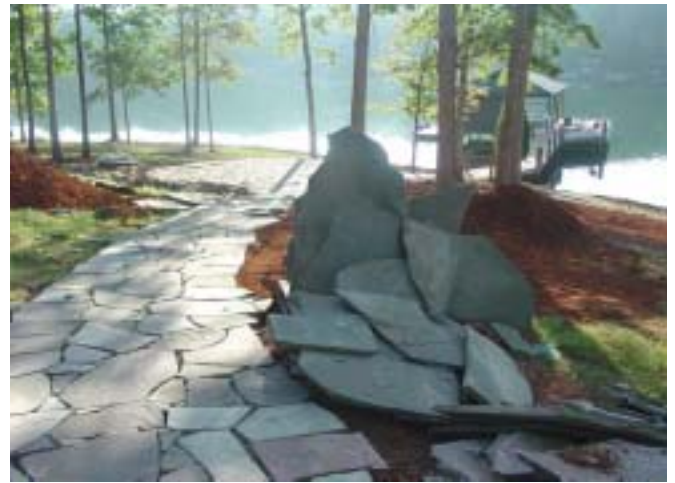
Work in progress: Stone walkway at Mascia home
